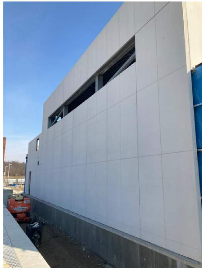
Faster enclosed buildings with windows installed at Stubbe's plant.
